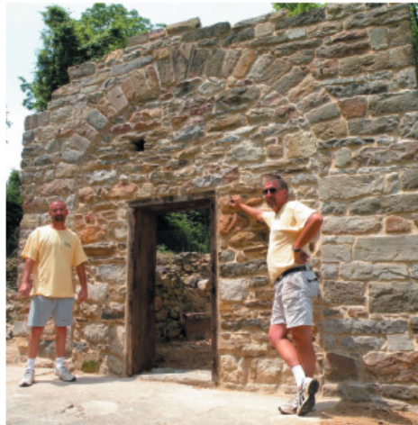
Ron Rickert (right) and his brother, Mike Rickert proudly show their work. The stone archway now looks spectacular with its new pointing work using Natural Hydraulic Lime.
