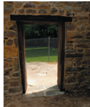
Below: It has now been stabilized by replacing the wooden frame and adding a new stone threshold.
